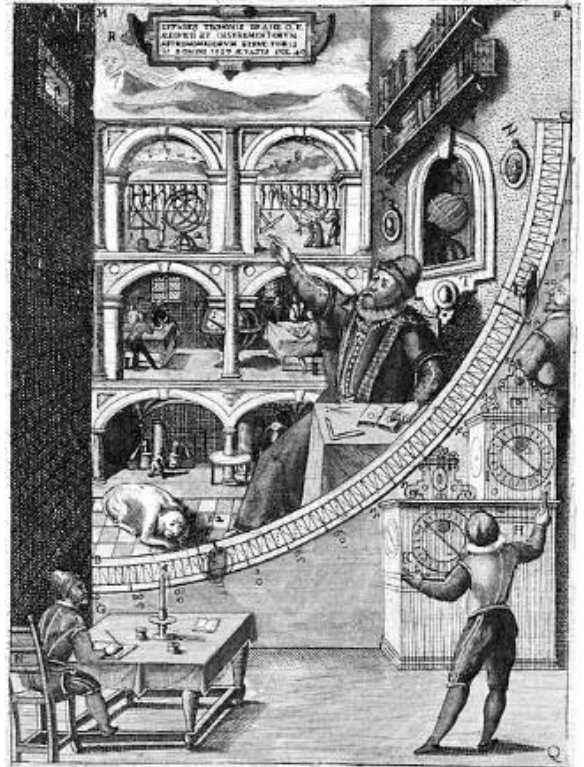
Figure 4: The large mural quadrant and small wall slit used to record star positions at Uraniborg
