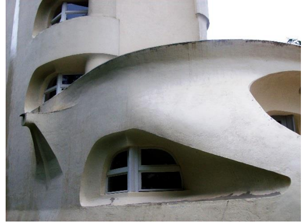
Figure 16: Detail of the Einstein Tower's window openings and scupper.
